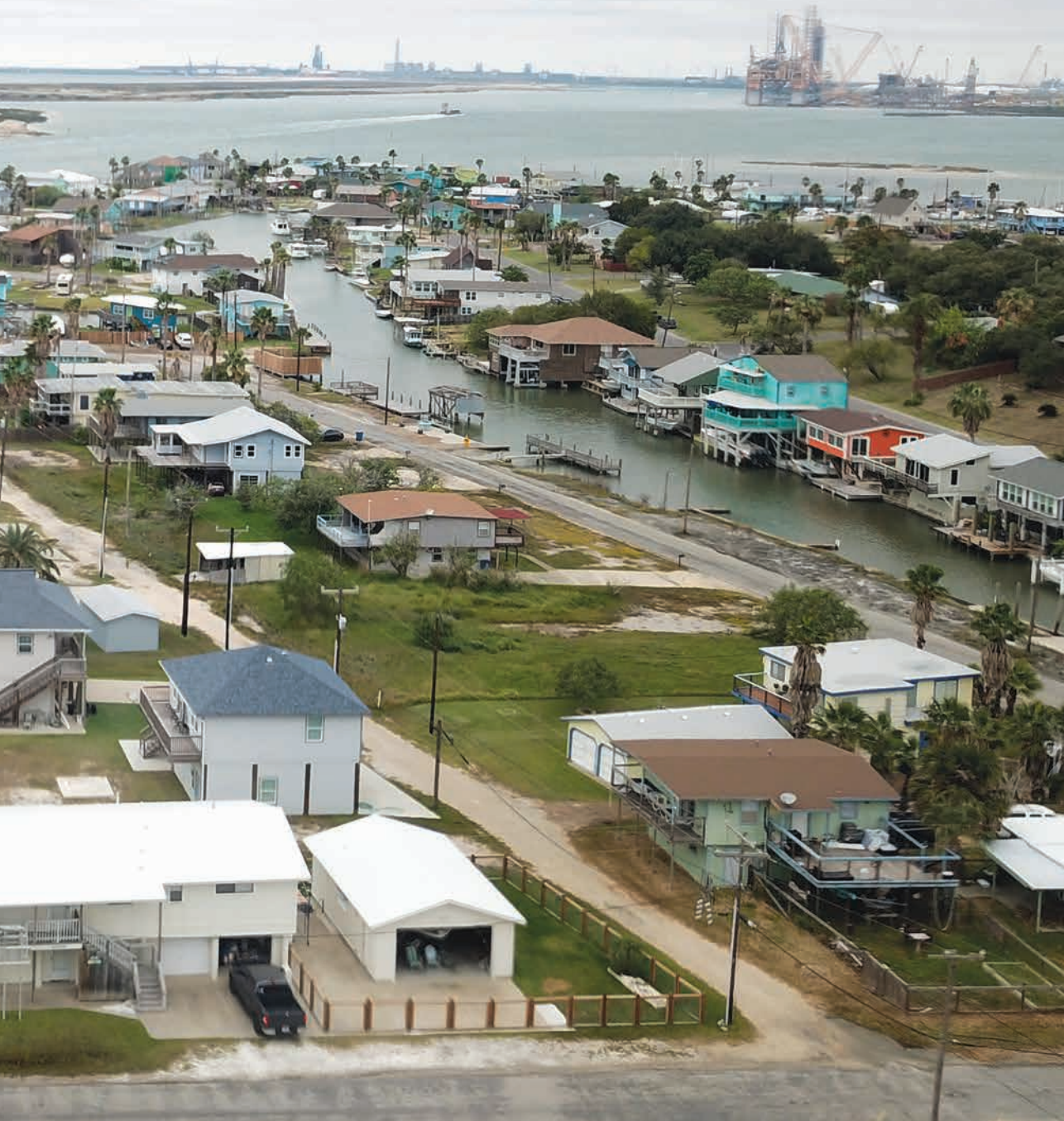
Figure 53. A coastal neighborhood located in Ingleside on the Bay in Texas, partly protected by a breakwater
