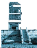
Coastal House Vung Tao, Vietnam Prana Architects 2010s
