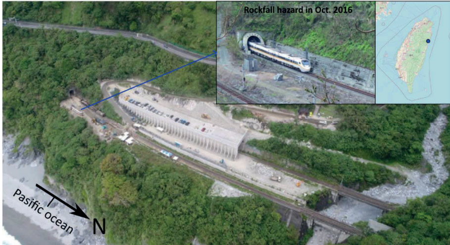
Figure 1: Study area (Shimizu Tunnel of the North-link railway line) for the current research.
