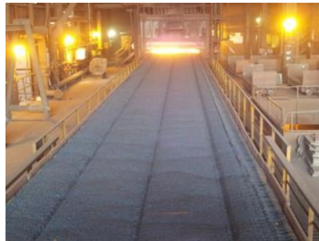
Iron ore sintering (Vanderbijlpark Steel Plant, South Africa)
