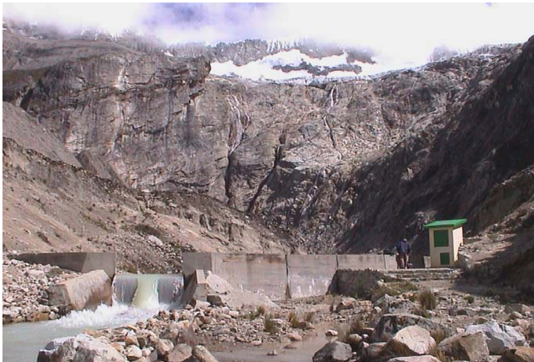
Figure 2.7: Runoff gauge at the outlet of Lake Artesococha (4200 m a.s.l.). Photo taken by Bernard Pouyaud.
