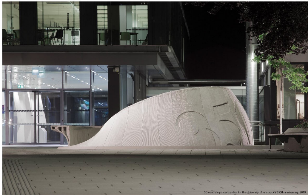
3D concrete printed pavilion for the University of Innsbruck's 350th anniversary 2019
