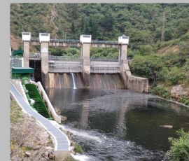
La Florida (7.5 MW) – Spain
